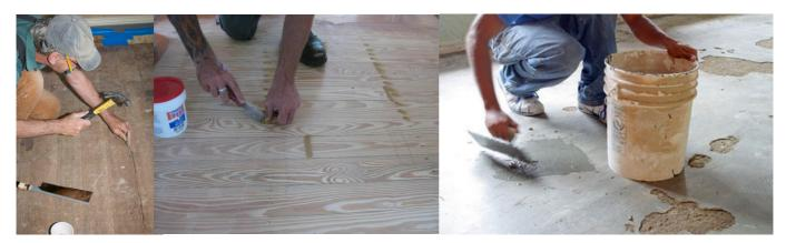
Fill any major holes and seal the surface of your floor if you will be applying floor leveller. This should be completed at this stage so you end up with the optimal fresh clean flat and level surface to begin your job.
