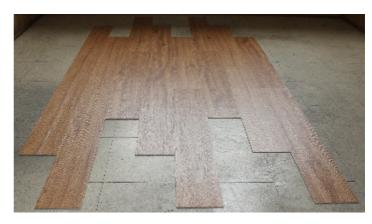
create different looks, for example offset by half, a third, or a quarter of a plank. The whole point is to mimic the look of floorboards. Just remember to always have at least 20cm of plank at each end of each row, 20 cm from joins surrounding your current plank joint, and plan out the width of your room so that both sides of the room have at least 9cm of plank width along the walls. This is to add stability to cut rows and planks and also to provide a move visually pleasing look to the room.
