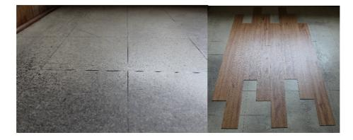
Again, it depends on the condition of the sub floor, if major damage is present, infill the major gaps and holes and level with floor leveller to get your final subfloor surface prepared for laying your new planks as outlined in the below steps.
