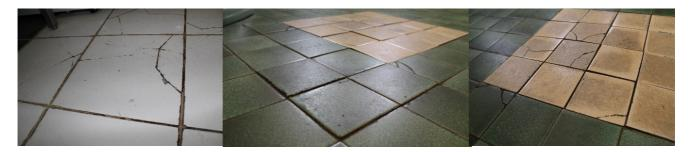
Once you have removed the imperfections, if you intend to apply a floor levelling compound, use a good quality ceramic tile sealer as this prepares the tiles for accepting a new layer above, and seals them to ensure they don't leach the Levelling compound into the ceramic tile, starving it from water and preventing it from setting correctly.
